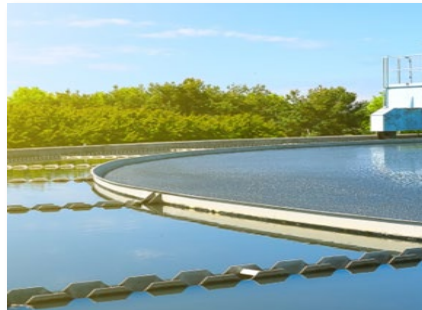
Specialized municipal and industrial water treatment
